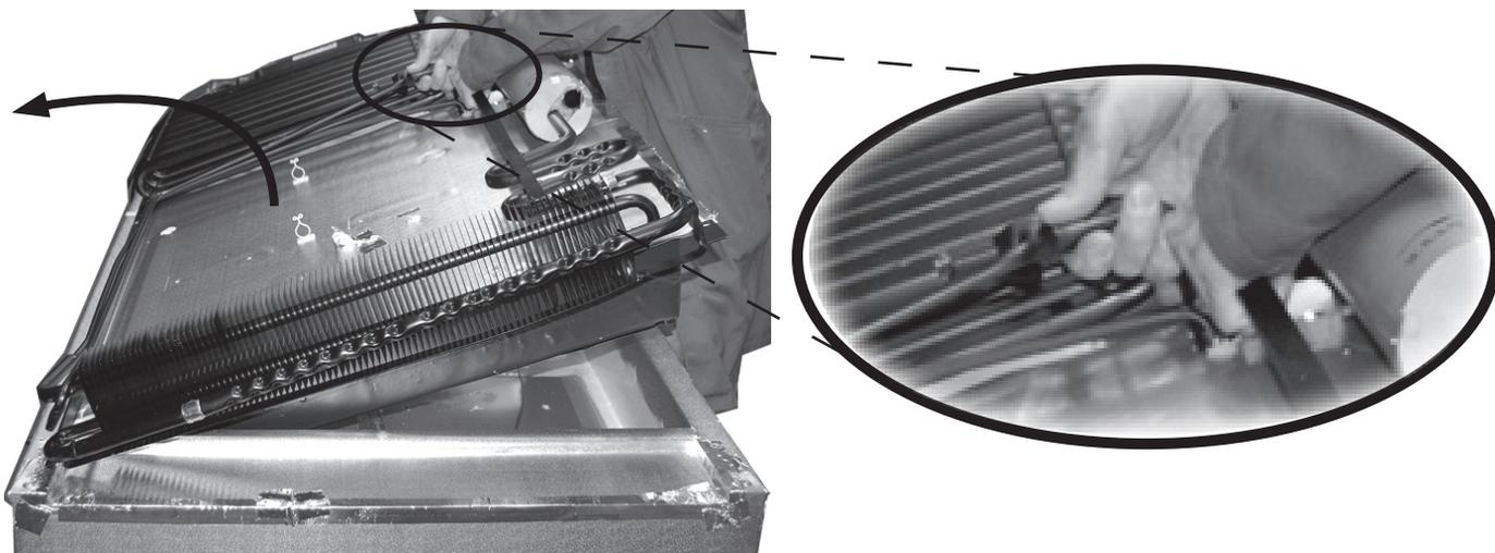
21. Locate the replacement cooling unit. Apply thermal mastic to the coils of the cooling unit.
