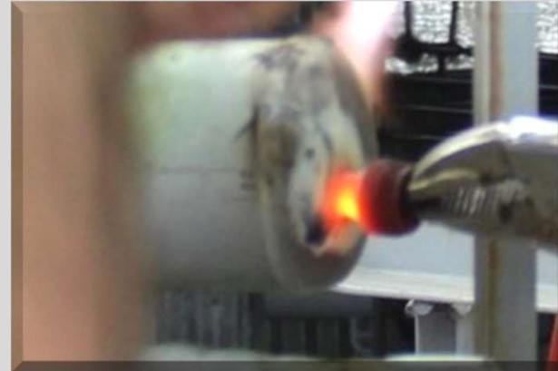
**6.1.8** With the torch on a low setting, heat the service valve behind the threads, making sure not to get on the threads.
