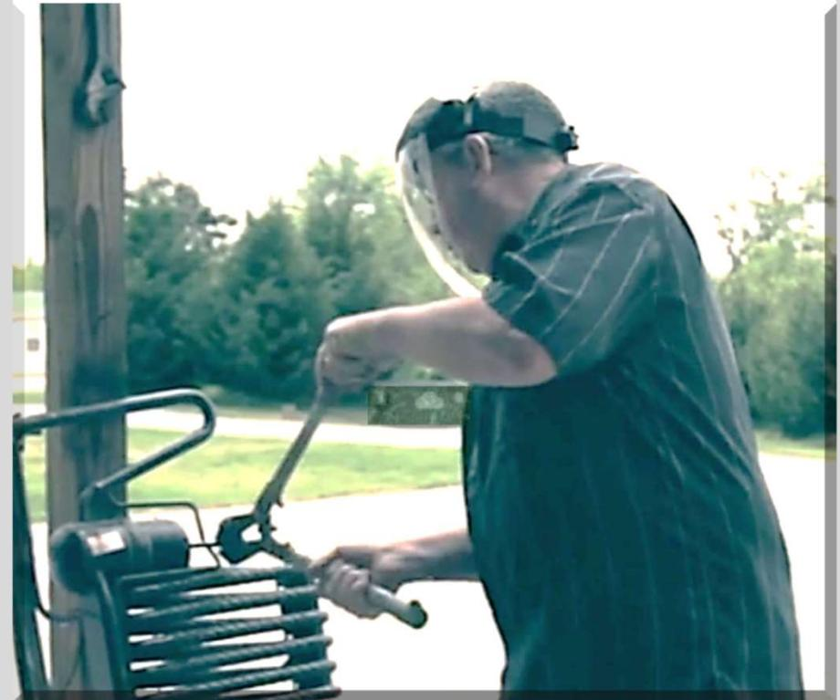
**22.2.4** With cutting wheel, cut the tip off where it was pinched together.
