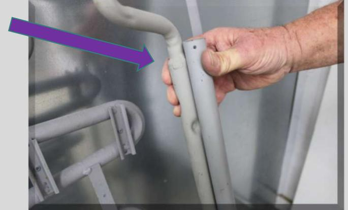
**20.1.3** It is also critical that insulation be properly installed between the back of the refrigerator cabinet and the boiler tube.
