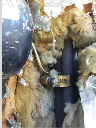
**20.1.5** Just add some extra fiberglass insulation on the backside of the boiler tube.
