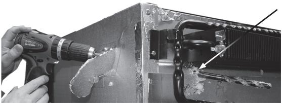
WATER SUPPLY HOSE Hole diameter 0,59" (15 mm)
