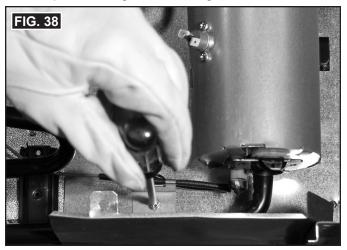
12. Reinstall three hex head drill point screws attaching cooling unit frame to refrigerator. Two screws at top, and one screw at bottom left. See FIG. 39.
