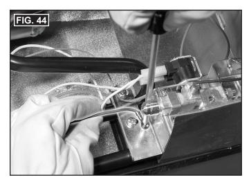
Connect wiring to the thermodisc on the flue jacket. This connection is not polarity sensitive.
